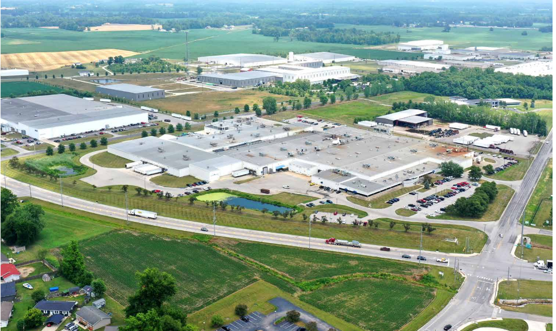
Drone photo by consultant team | June 2023
