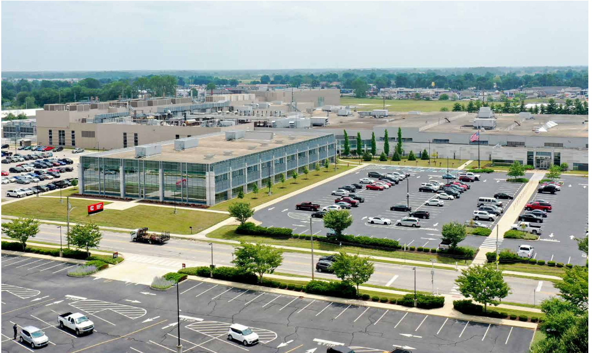
Drone photo by consultant team | June 2023
