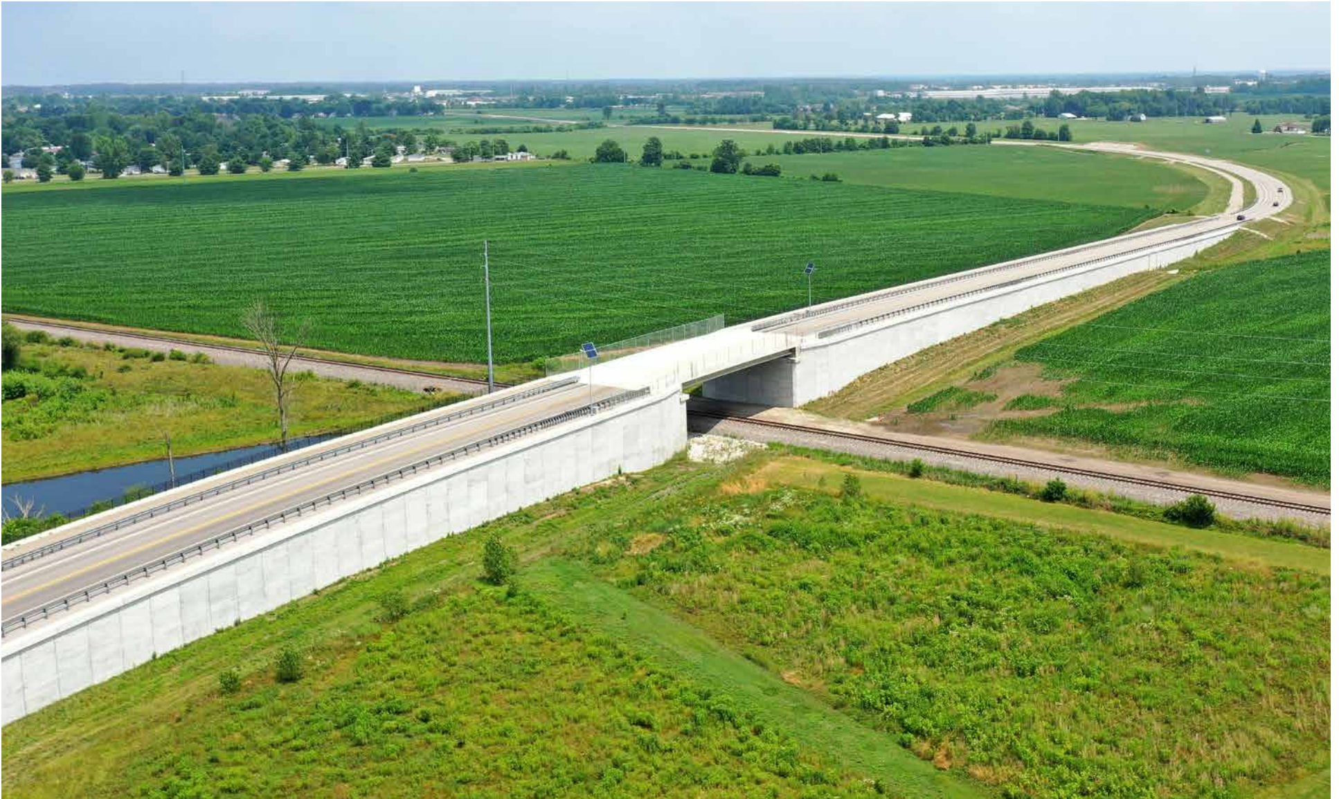
Drone photo by consultant team | June 2023
